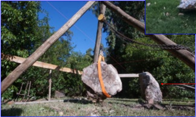
→ We created a secondary structure to move and locate the rocks.
